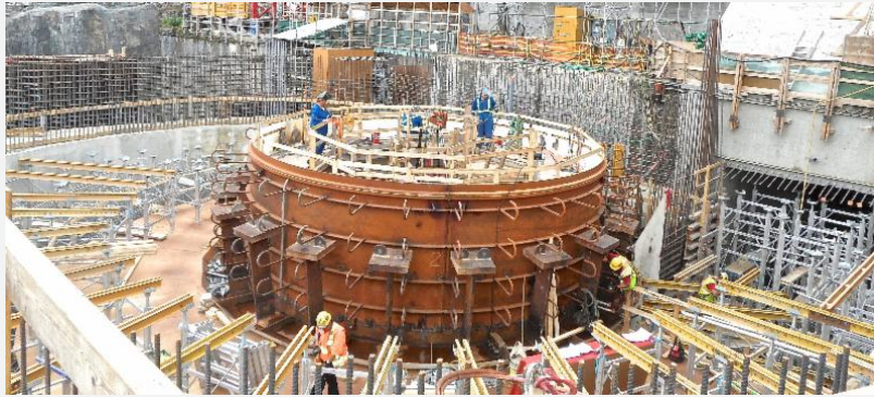
Kipling G-3 unit scroll case hoarding and discharge cone prior to concrete pouring
