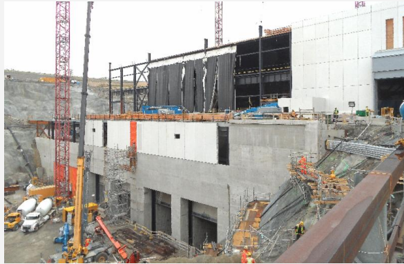
Smoky Falls 2 powerhouse and tailrace (dewatered)
