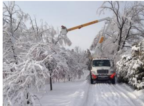
PWU Workers from PowerStream work to restore power.
