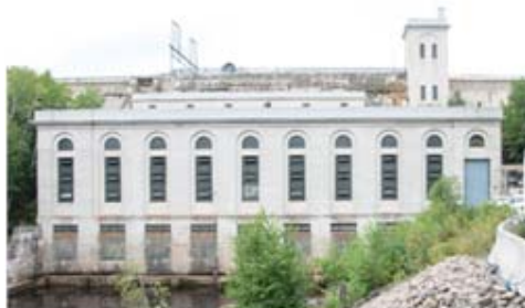
The original Smoky Falls GS that is being decommissioned
