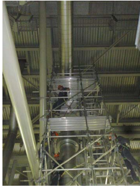
OPG Darlington Scaffolding Submitted by: Paul Robichaud
