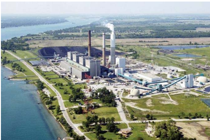
Photo: Lambton Generating Station
